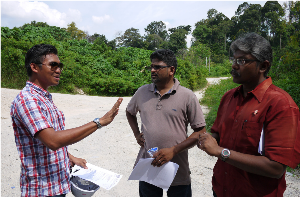
Executive Director of SUARAM, Sevan Doraisamy (centre) and PSM Secretary General, A. Sivarajan (right) speaking with TNB contractor on the construction of Cheras Hartamas Pylon
